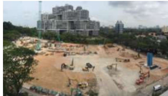
Phase 2: Completed demolition works
