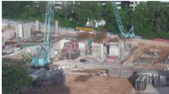
Phase 1: Superstructure works in progress
